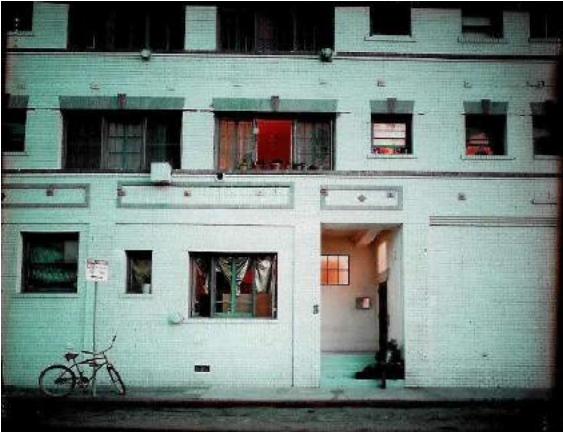
© Cheryl Himmelstein and the Los Angeles Public Library. The Fenmar Apartments Bldg. on Brooks Ave., a few months before it was seriously damaged in a huge fire. Taken between July 2002 and August 2003 as part of the Los Angeles Public Library's Neighborhood Project. [This, and other photographs, are in color in the online edition of Views.—Ed.]
