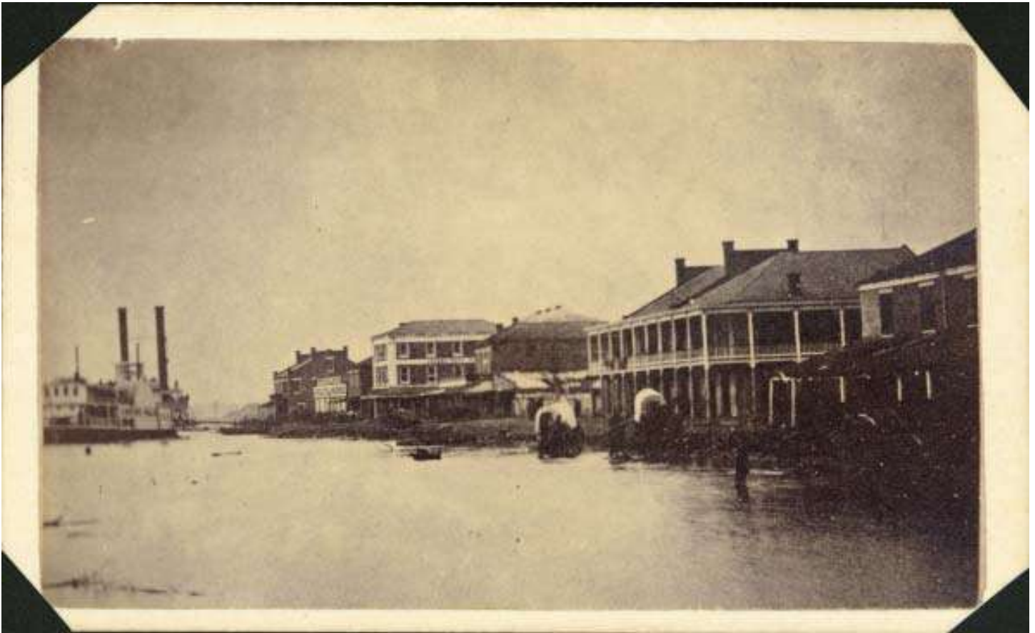
High water at the levee, Baton Rouge. One may see in the image that there is no levee. Tide lines are visible on the buildings to the right of the wagons. The steamboat is the "Empire City," which served as headquarters for Federal army commanders while Baton Rouge was occupied. Marshall Dunham Photographic Album (Mss. 32410109), Louisiana and Lower Mississippi Valley Collections, LSU Libraries, Baton Rouge, Louisiana, USA. Mark Martin's remarks about this amazing album begin on p. 17.
